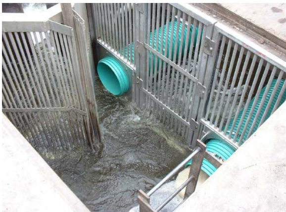
Resistivity counter tubes in the trap cell of the Bonaparte Fishway
