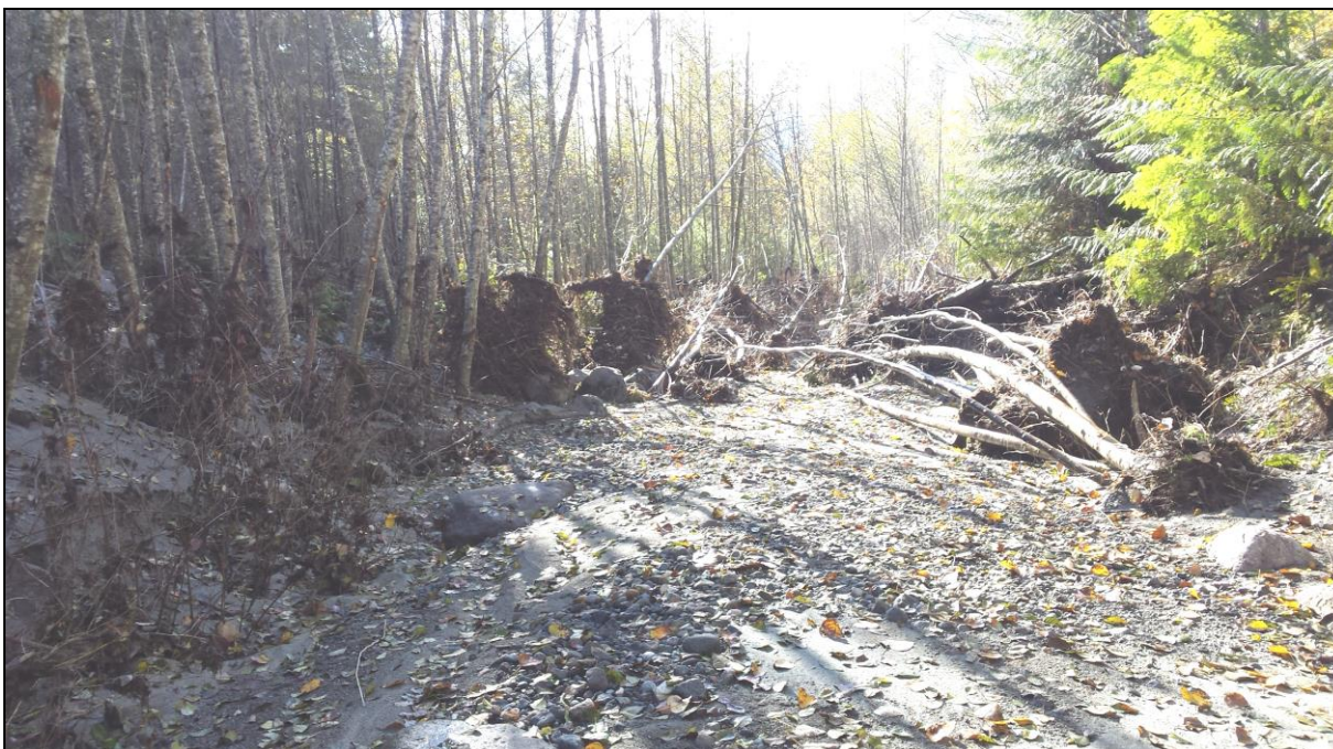
Figure 4: Looking downstream of the berm showing the damage caused when heightened flows from the Squamish River mainstem overtopped the protective berm built in 1994. Despite many trees being pushed over and fine sediment accumulating in depositional areas, the channel survived relatively well with no significant structural weaknesses observed.
