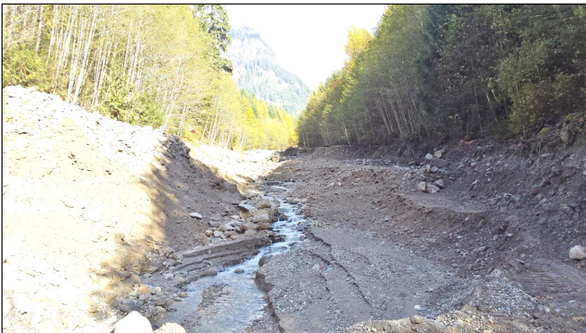
Figure 7: Photo looking upstream from the repaired road crossing where Turbid Creek took out the culvert and road in a significant earth-moving, debris torrent. Some of the bigger rocks transported in the event exceeded 6 feet in diameter. Photo taken after much debris had already been removed with an excavator.
