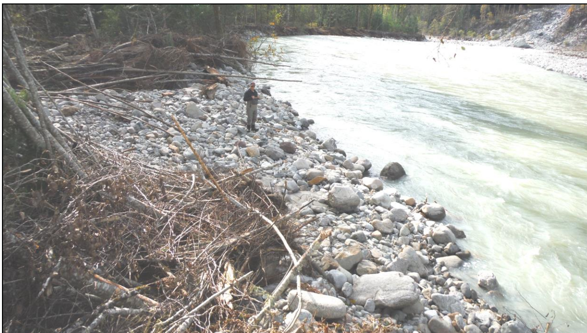
Figure 3: Looking downstream on the Squamish River mainstem showing the gap (exposed rocks) remaining after the high water event over-topped the gravel berm (out of photo to the left).
